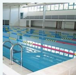
Piscina Municipal de Azambuja - Interior
