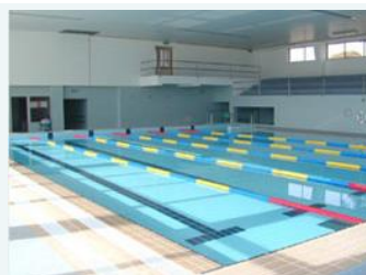
Piscina Municipal - Tanque interior
